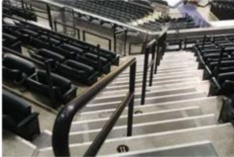
Picture shows example of preferred handrail design. Note: Stainless steel required
